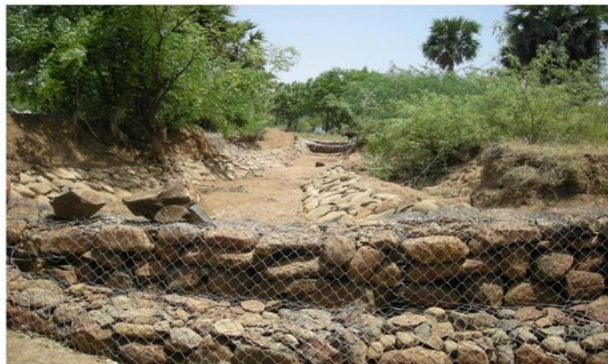
Plate 3.2: Gabion Check Dam to counter erosion
