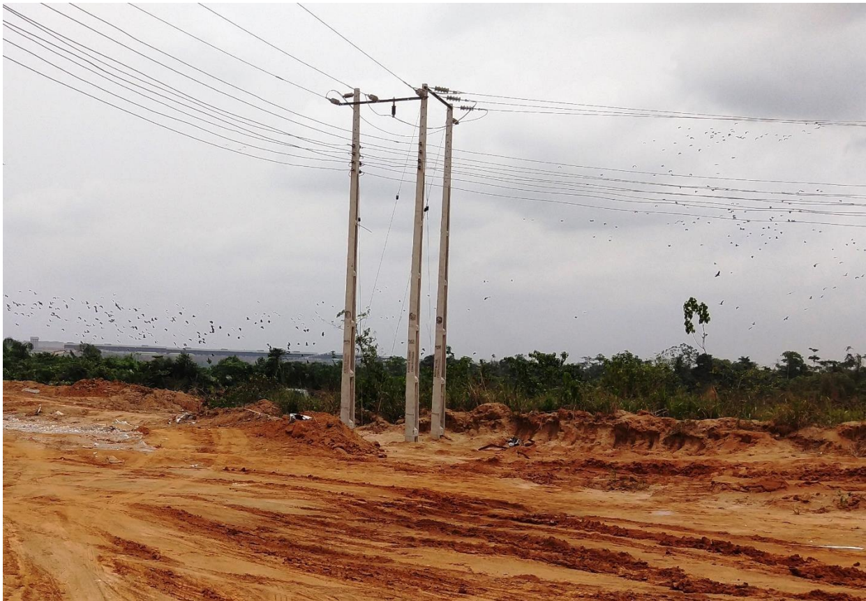
Plate 3.2: Power transmission lines in the City
