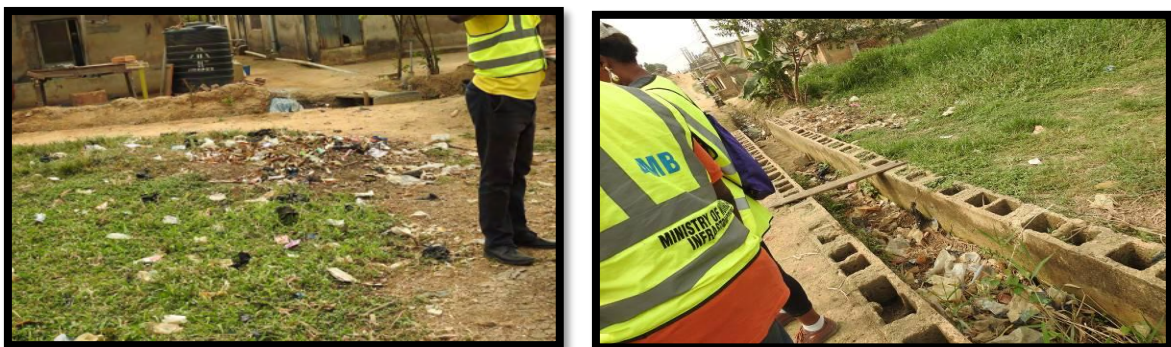
Plate 3.18: Waste Disposal and Drainage Facilities in Ori-Okuta
