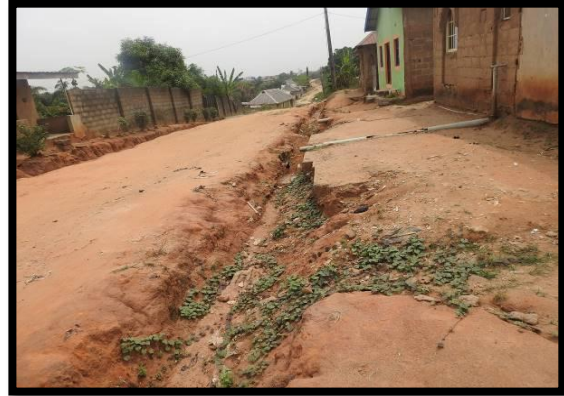
Plate 3.19: Waste Disposal and Drainage Channel Affected by Erosion in Tapa, Island
