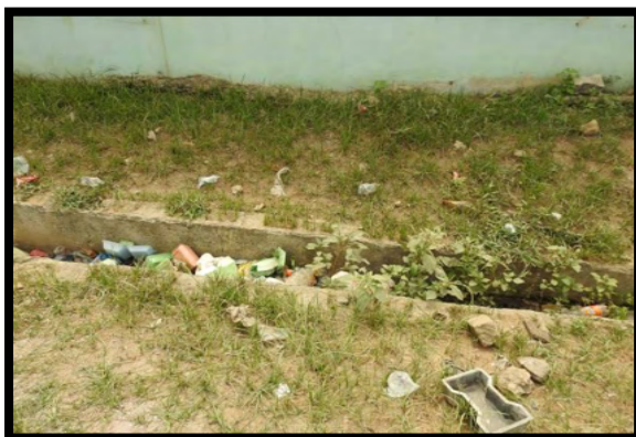
Plate 3.8: Clogged Drainage Channels with Waste and Vegetation (Grasses) around Sparklight Estate
