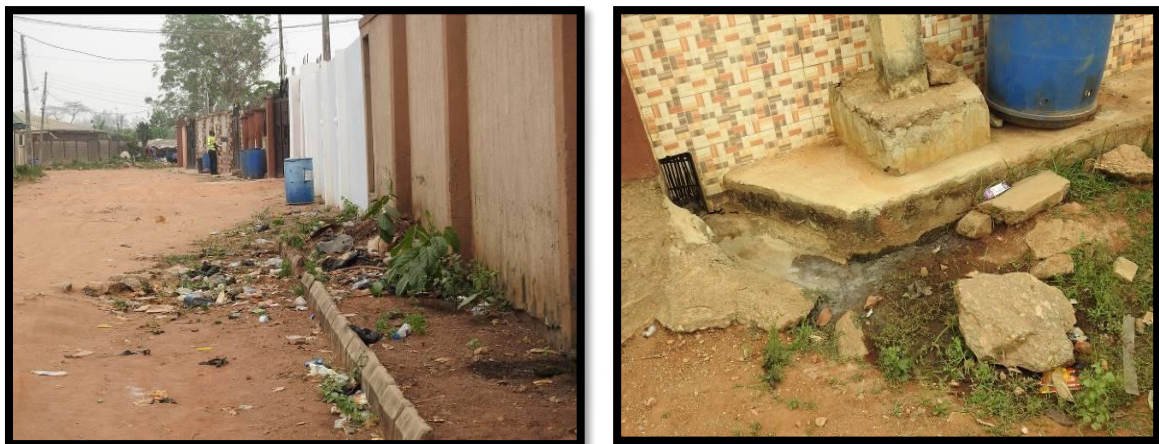
Plate 3.24: Waste Disposal and Drainage Facilities in Oku- Adebo
