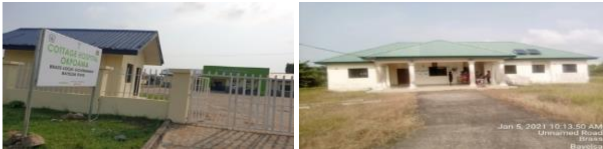
Plate 4.35: Typical of Cottage Hospital and Primary Health Center in Brass Island Shipyard project study communities
