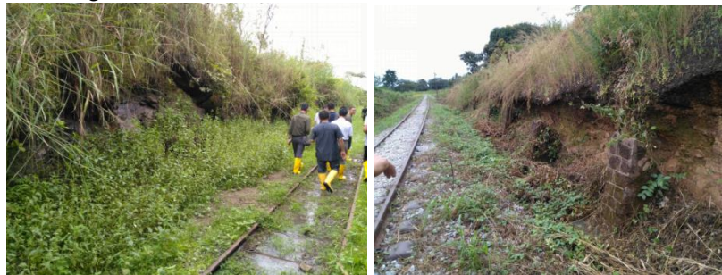
Plate 2.3: Collapsed at cutting
