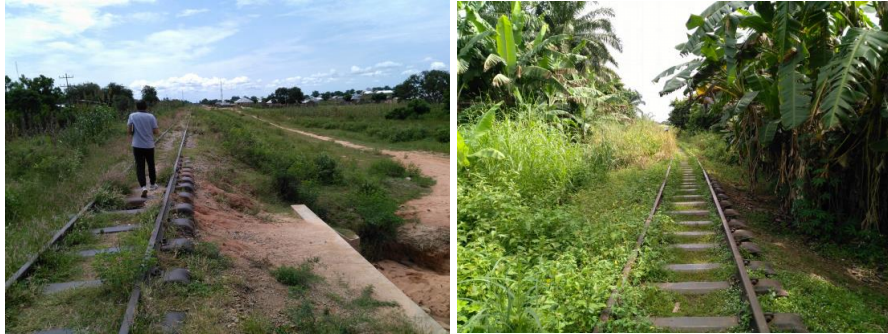
Plate 2.1: insufficient of shoulder width
