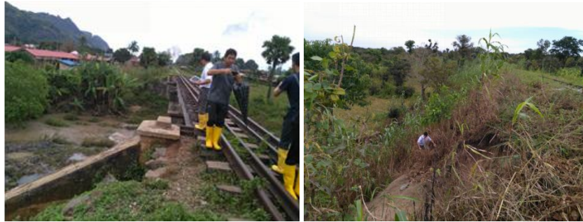
Plate 2.4: Slides and collapses in transition section between bridge and embankment
