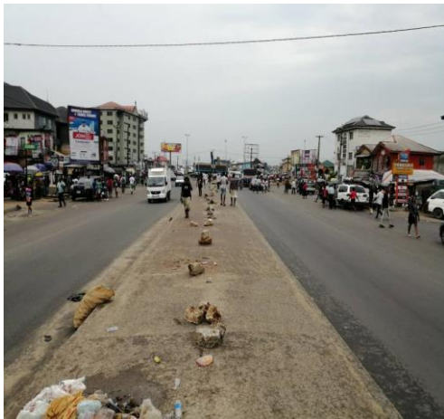
Plate 4.29: Road infrastructure in Port Harcourt metropolis
