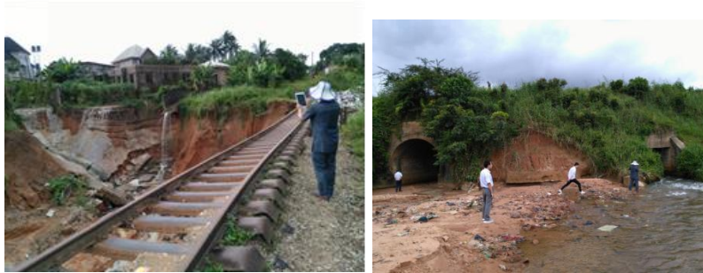
Plate 2.2: Subgrade destroyed and collapsed by flood
