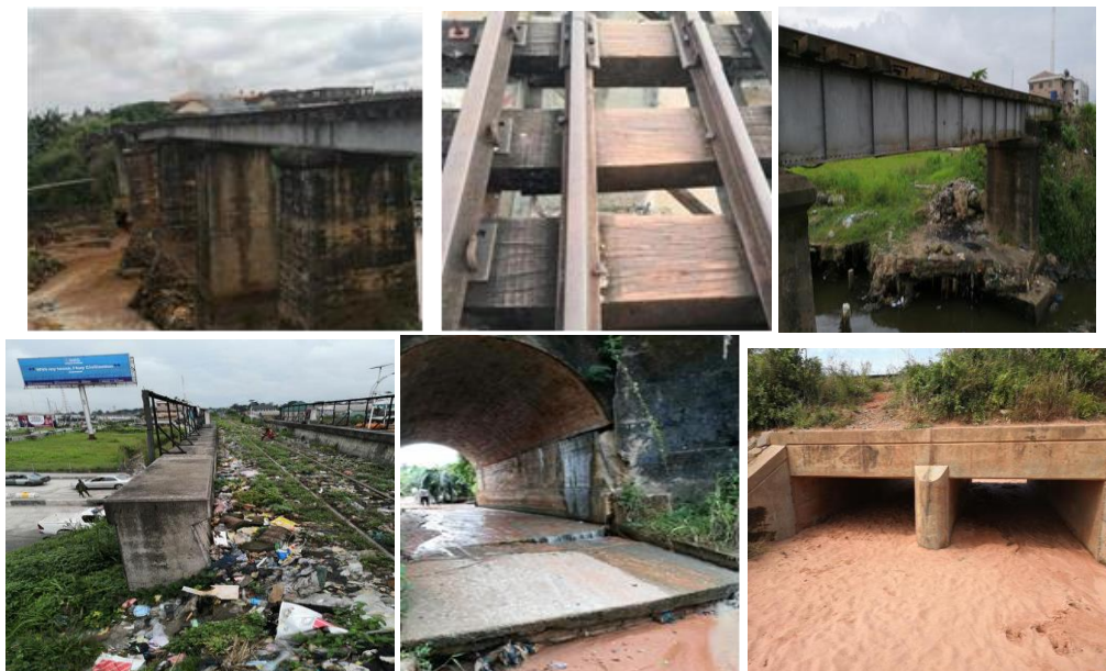
Plate 2.5: Serious damages on bridge and culvert structures
