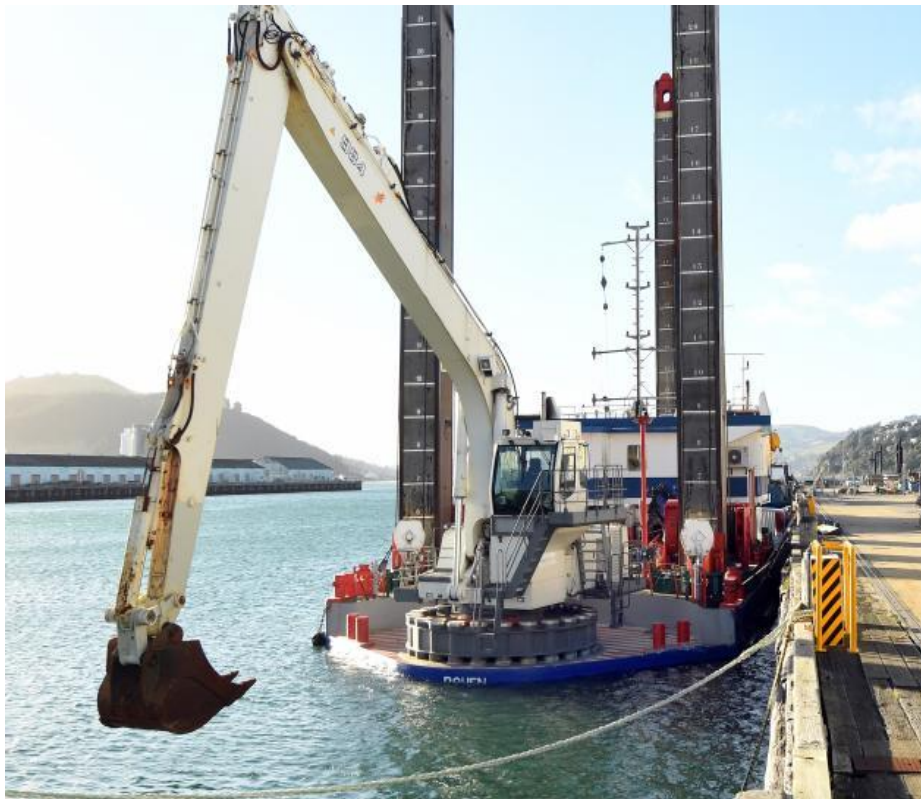
Figure 3.7: Back Hole Dredger (BHD)
