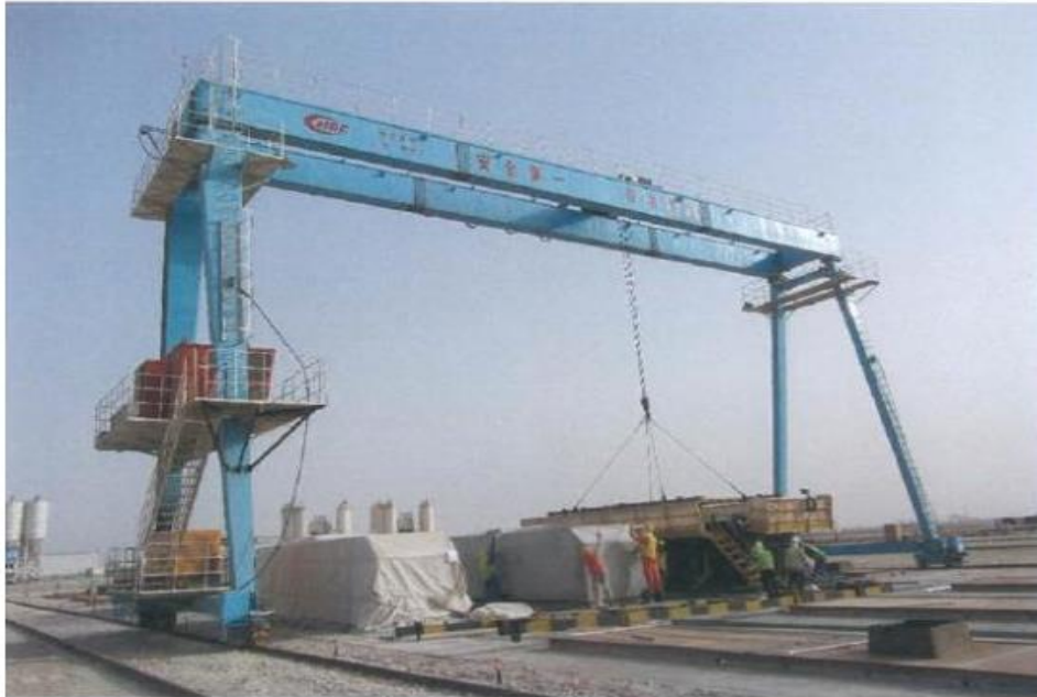
Figure 3.11: Gantry Crane in Fabrication Yard
