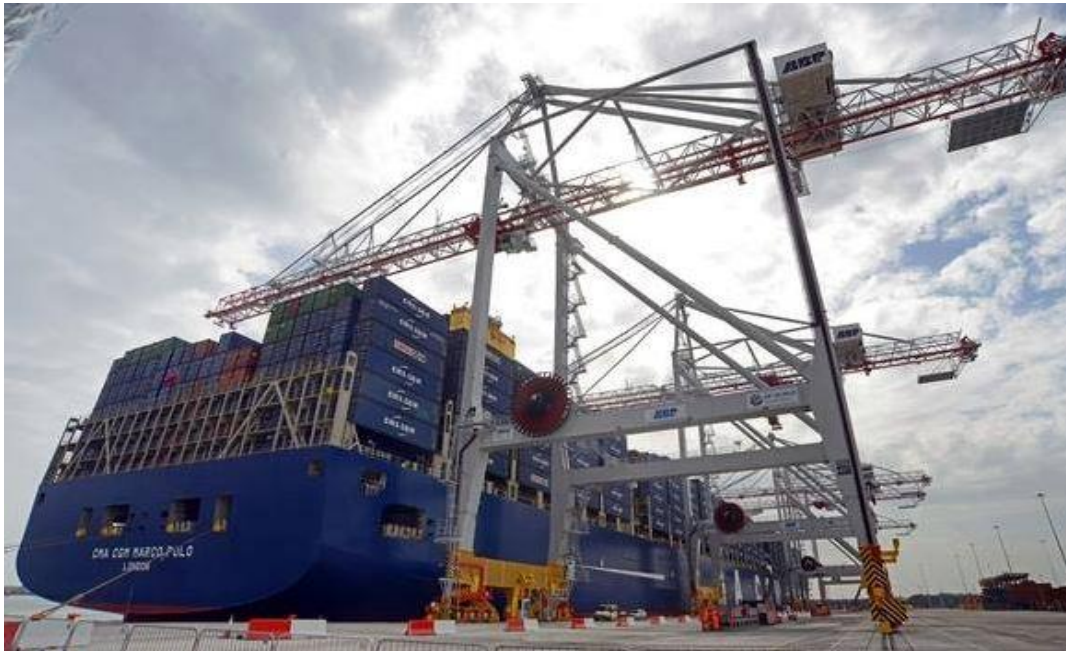
Figure 3.10: A typical container berth
