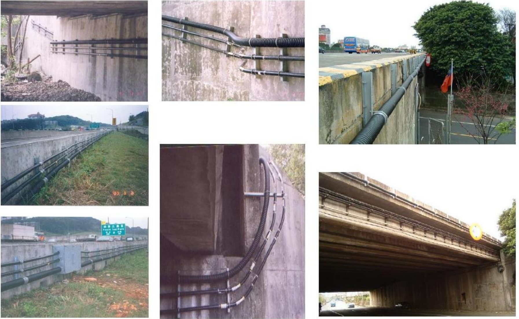
Plate 3.4: Laying of Optic Fibre across the bridge
