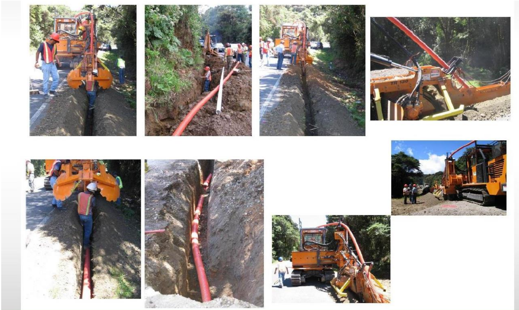
Plate 3.3: Laying of Optic Fibre along highway
