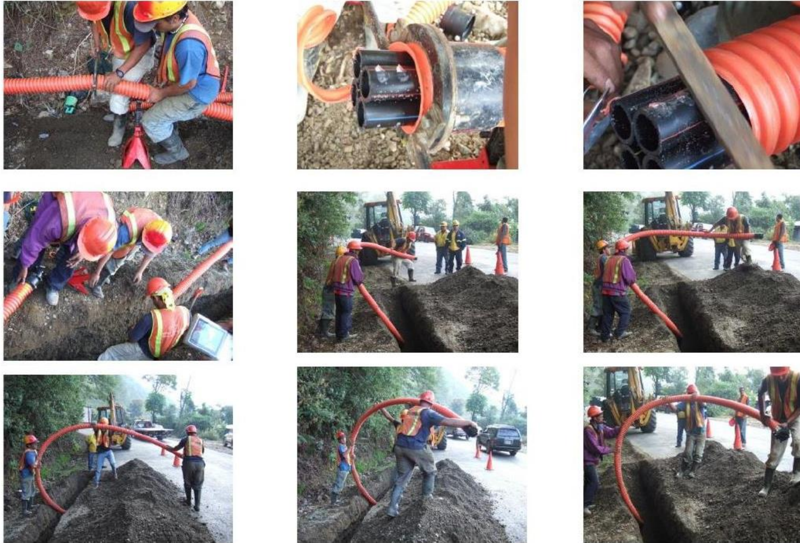
Plate 3.5: Laying of Optic Fibre along Mountain area
