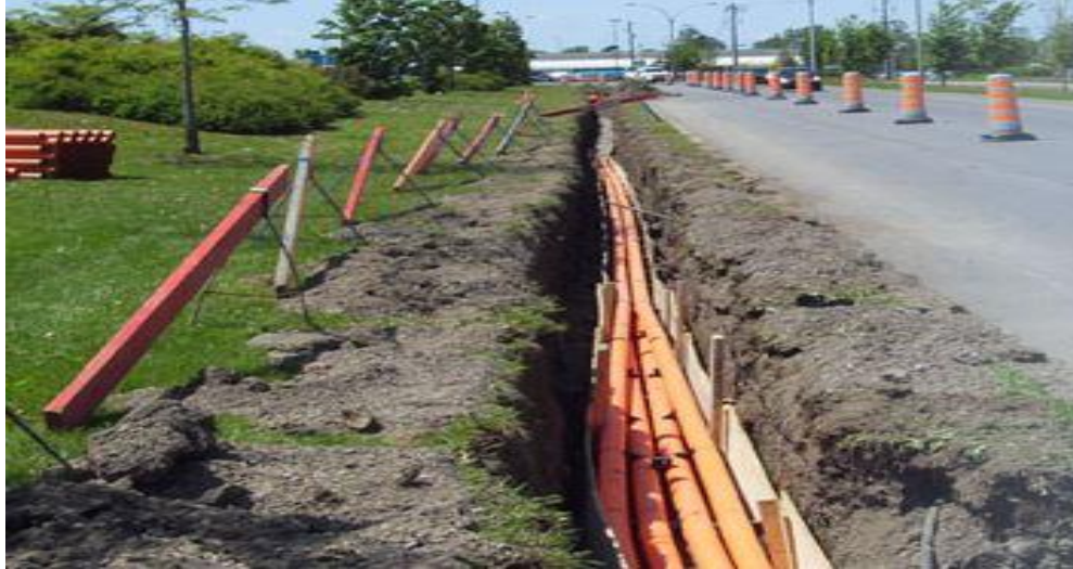
Plate 3.2: Typical Cable ducts in open trench
