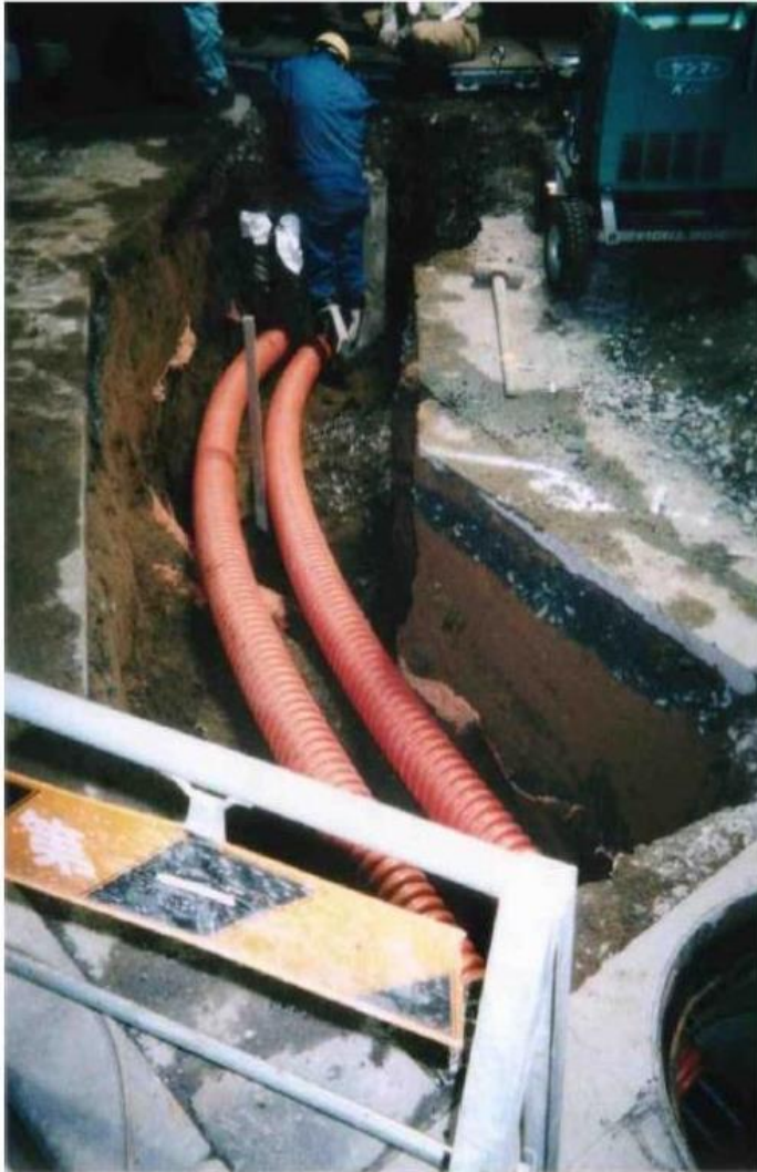
Plate 3.7: Installation of Curved Manhole for Optic Fibre
