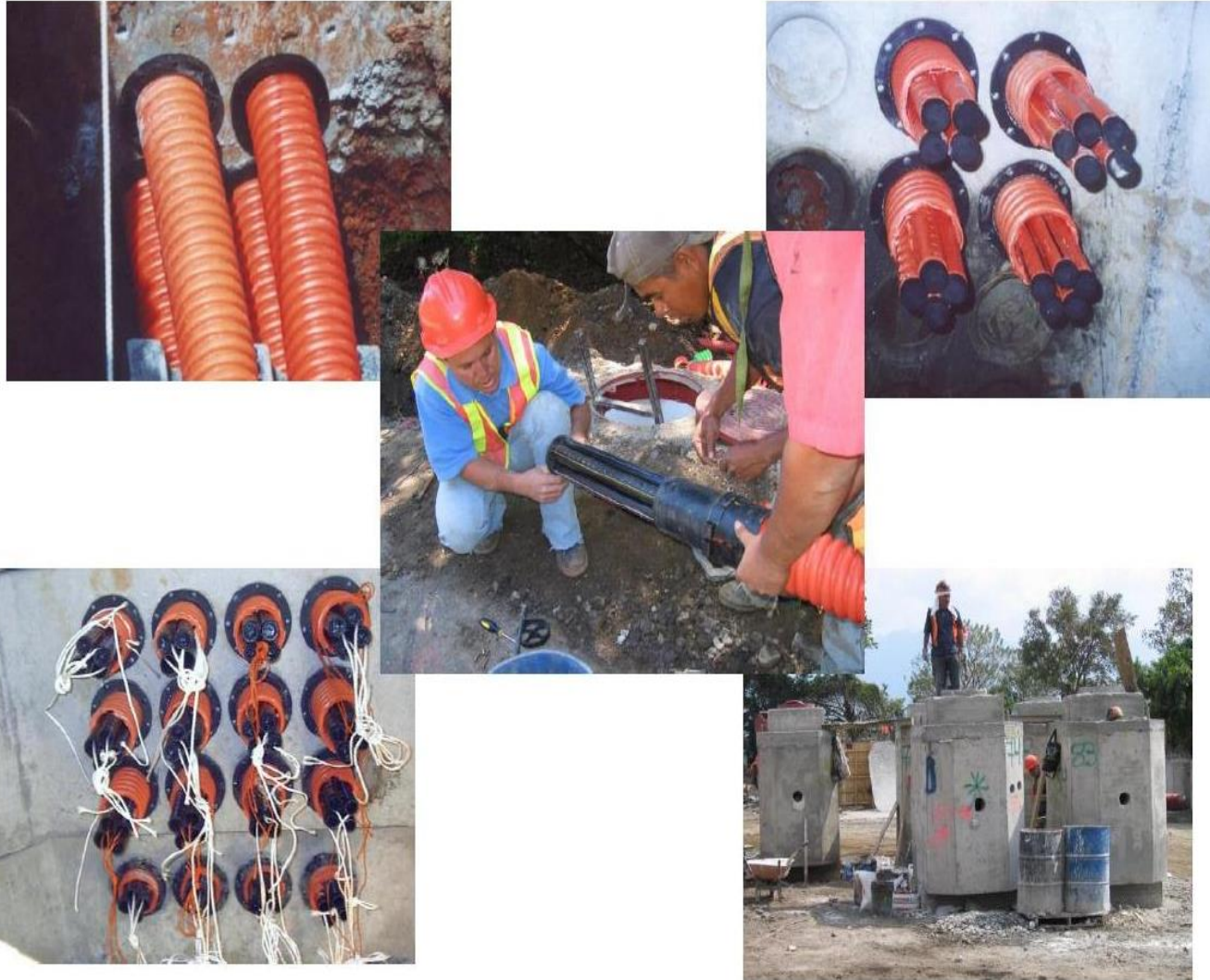
Plate 3.6: Installation of Optic Fibre Manhole
