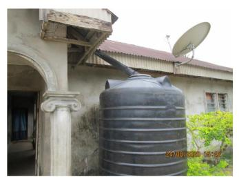
PLATE 4.29C: WATER TANK INSTALLED TO COLLECT RAIN IN POLAKU COMMUNITY
