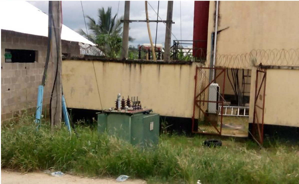
Plate 4.28: A transformer station supplying PHCN electricity to Tunama residence
