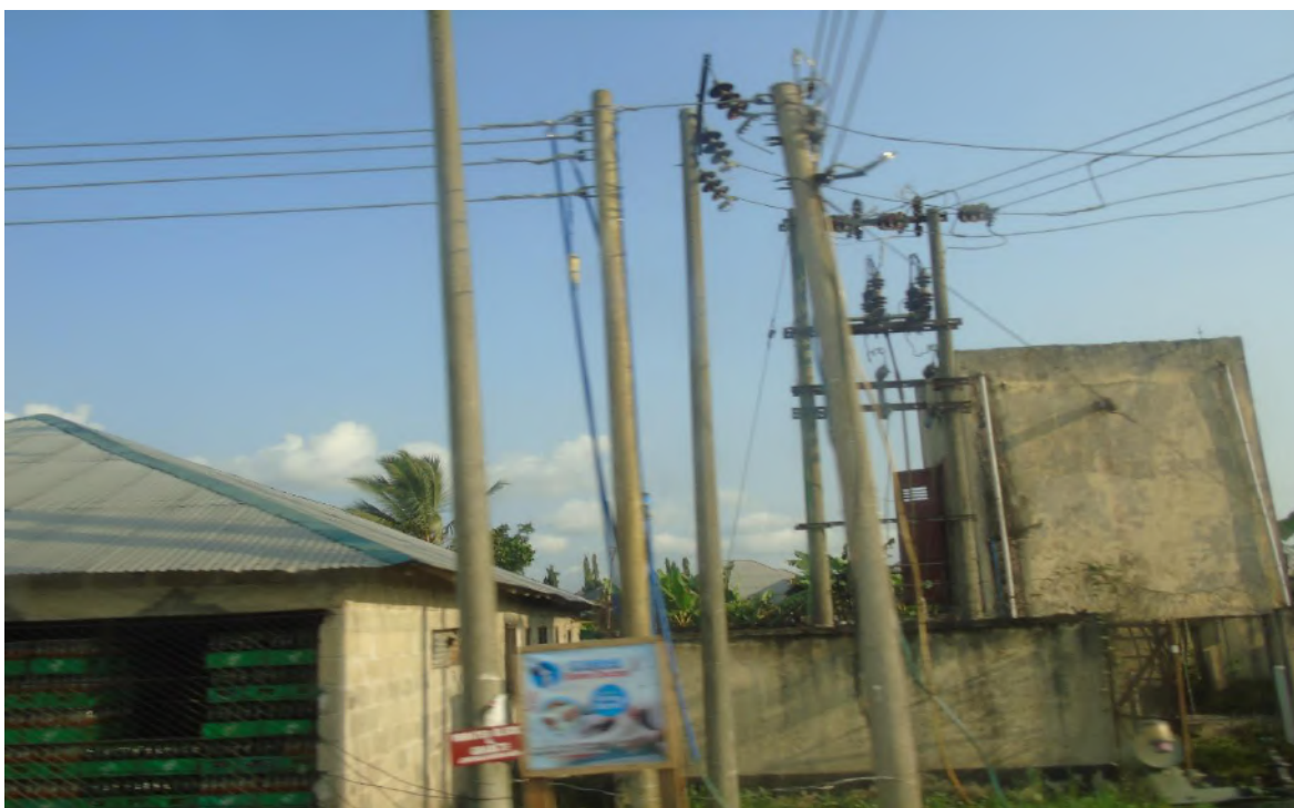
Plate 4.27: Distribution lines on concrete poles at Tunama community
