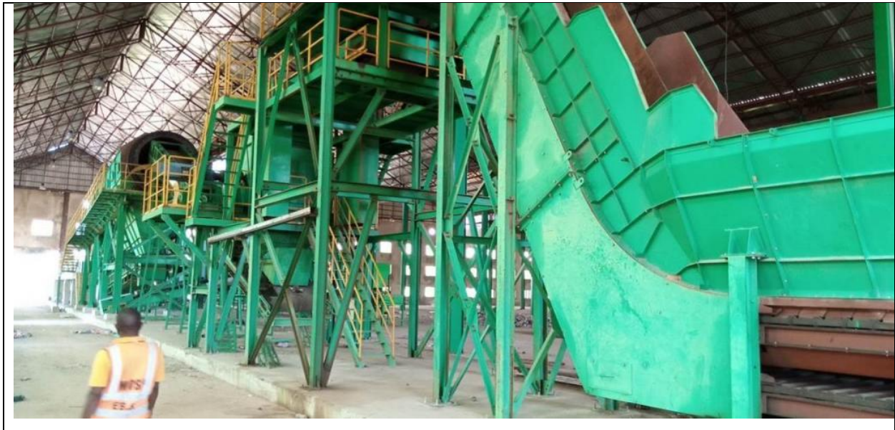
Plate 4.27: Ebonyi Waste Pulverisation Plant at Umuoghara
