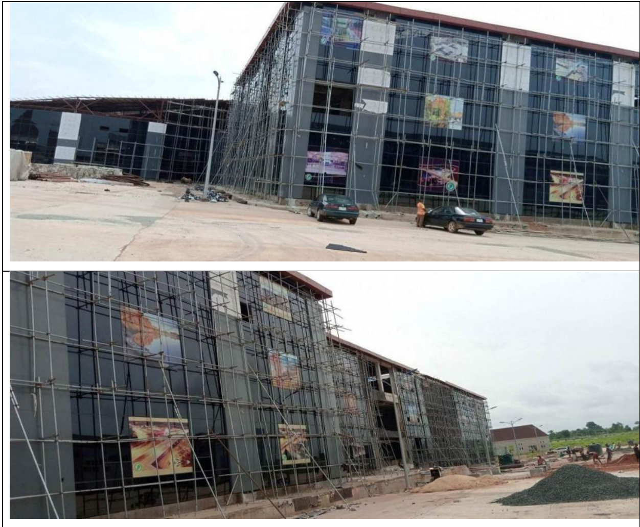
Plate 4.18: Shopping Mall nearing Completion
