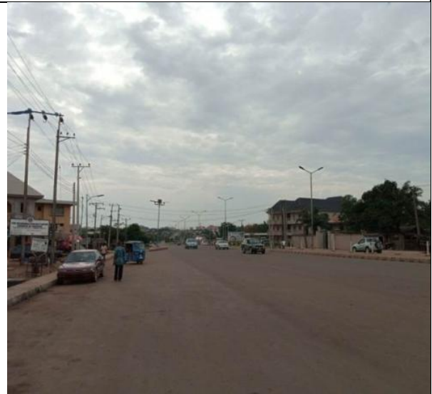
Abakaliki – Enugu Expressway
