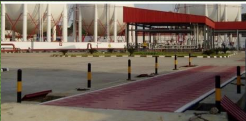
Figure 3.2E: View of SEL LPG Facility Weigh Bridge
