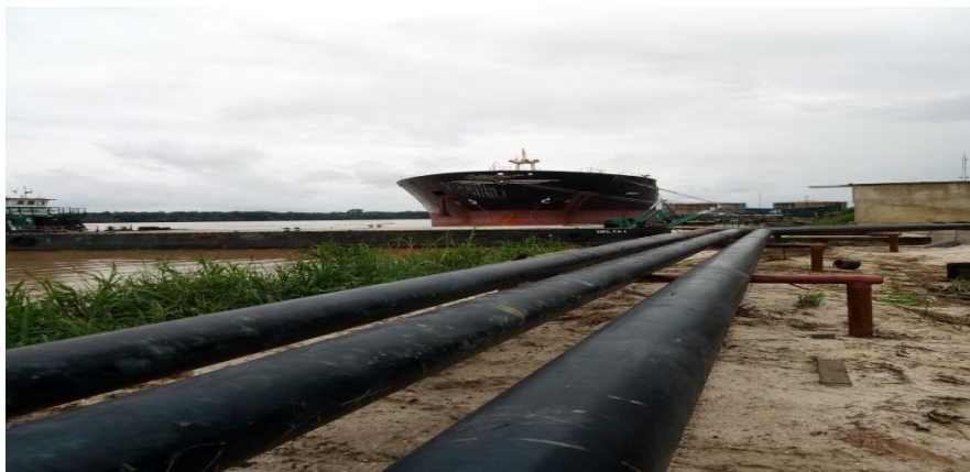
Plate 4.46: Tank farm sites with heavy pipes for transporting refined crude products
