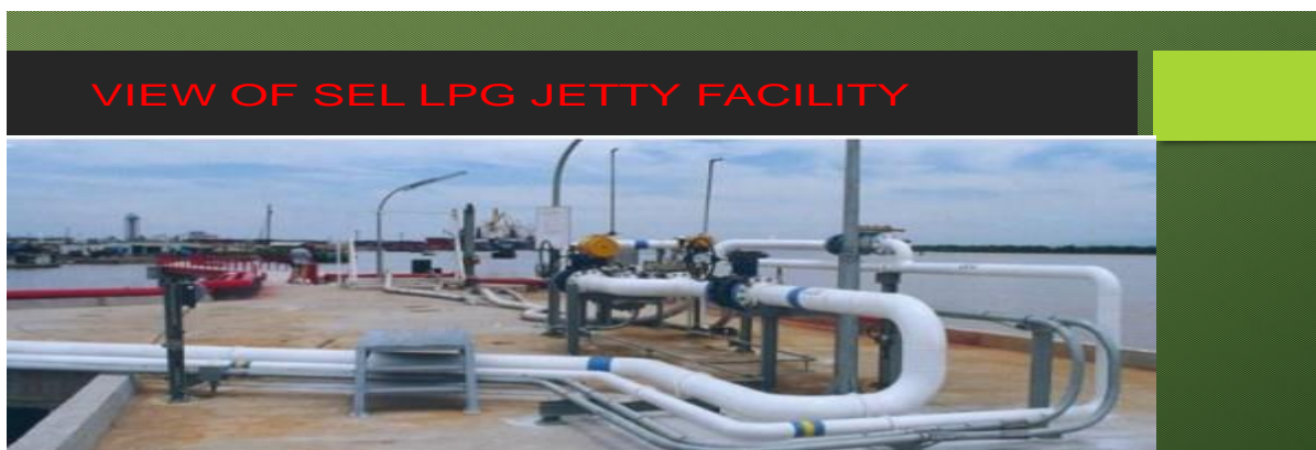
Figure 3.2C: View of SEL LPG Facility Equipment
