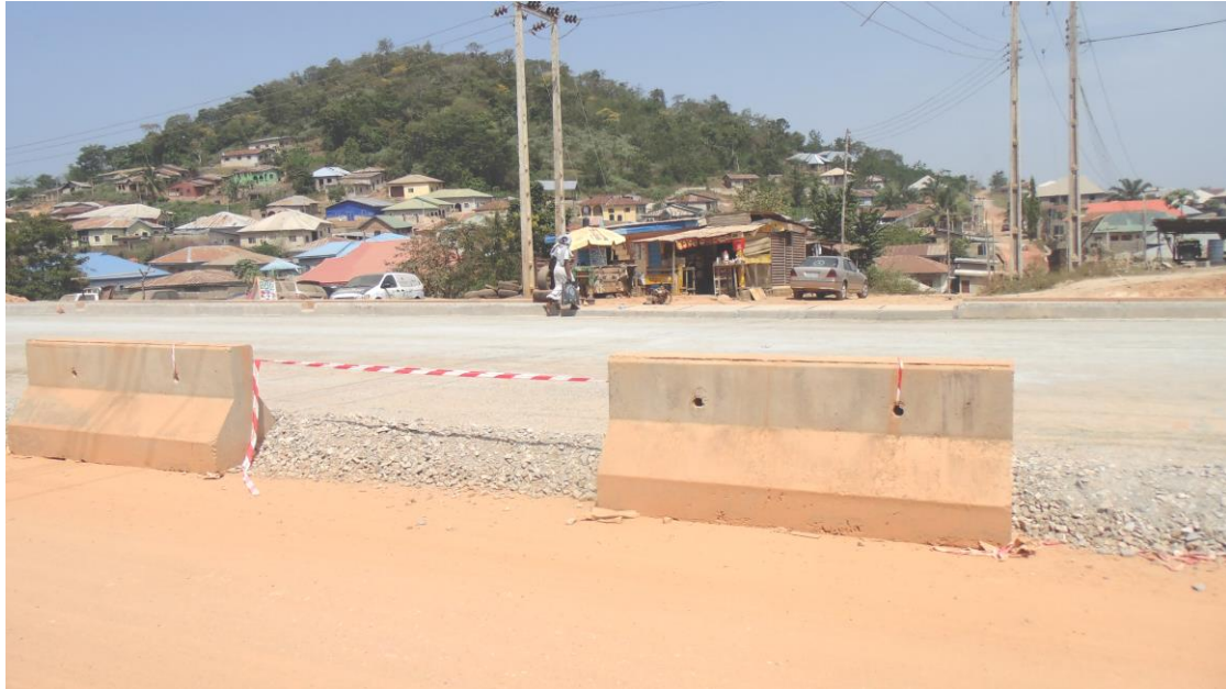
Plate 3.4: Section II between NTA road junction and Ofin Village
