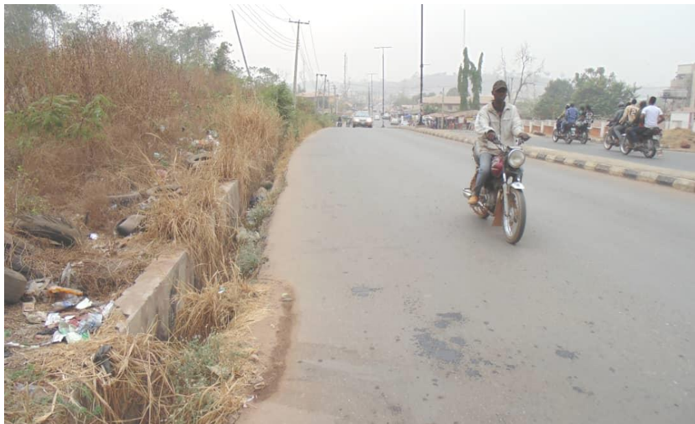
Plate 2.3: Drains covered with vegetation
