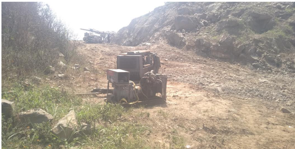
Plate 2.2a and 2.2b showing sections of the road with rocky terrain
