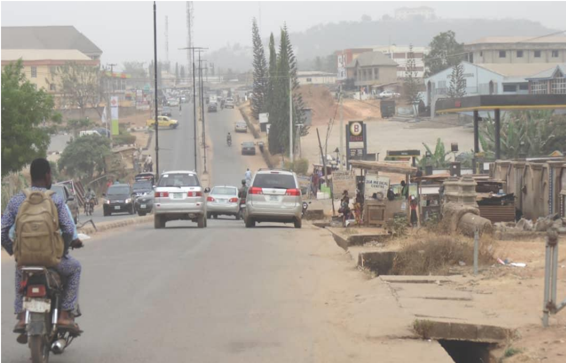
Plate 3.8: A section of Bank road with built up areas on both sides of the road.
