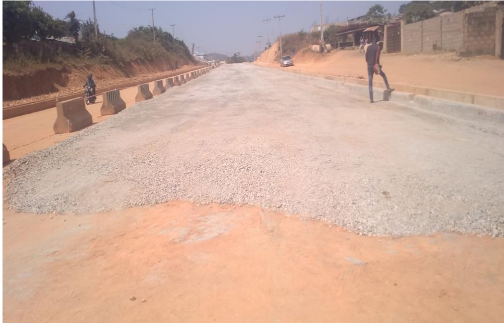
Plate 2.1 The New Ado –Iyin road at the state pavilion, Ado Ekiti
