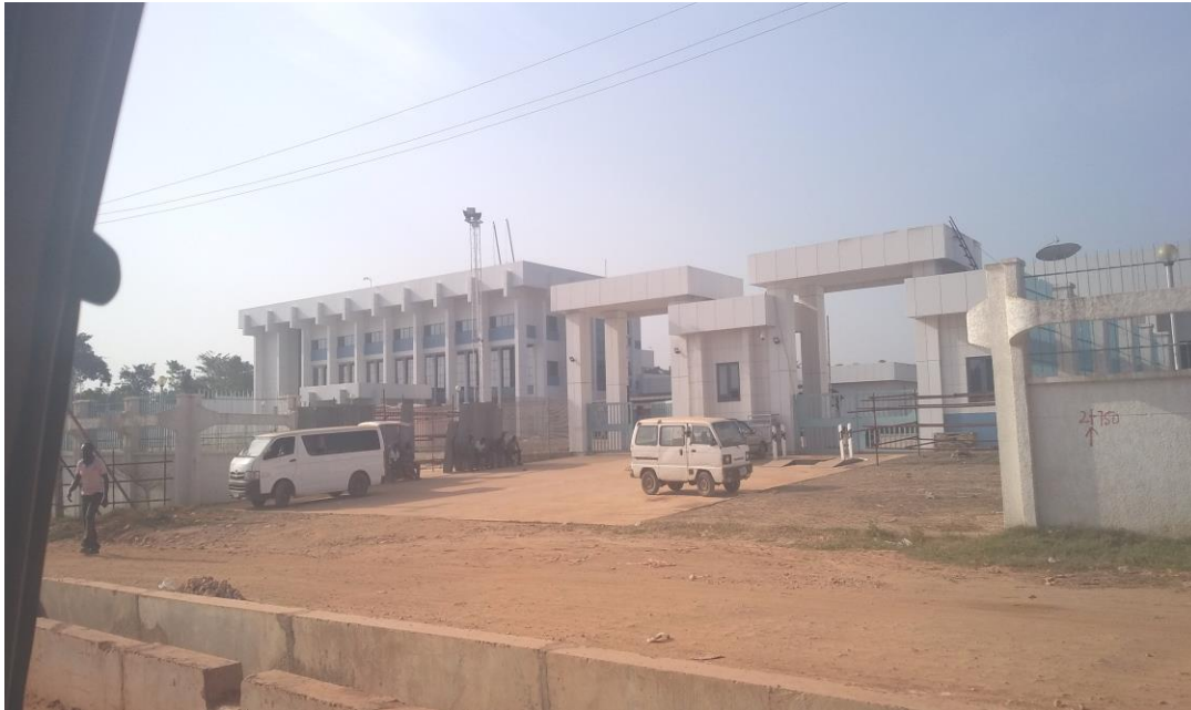
Plate 3.9: New Central bank building along the project area
