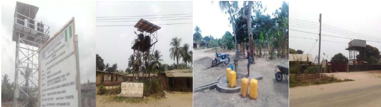
Plate 4.20: Water facilities at Igbuku, Emu-Iyasele and Ashaka by EU, MPP3 and Delta State government respectively aimed at achieving MDG goal of increasing access to improved drinking water
