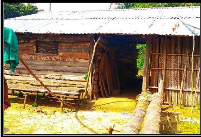
Plate 4.68: A newly constructed residential Building in the Area
