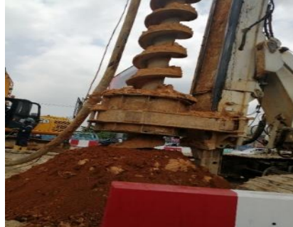
Plate 4.3: Geotechnical investigations at Rumuola Junction
