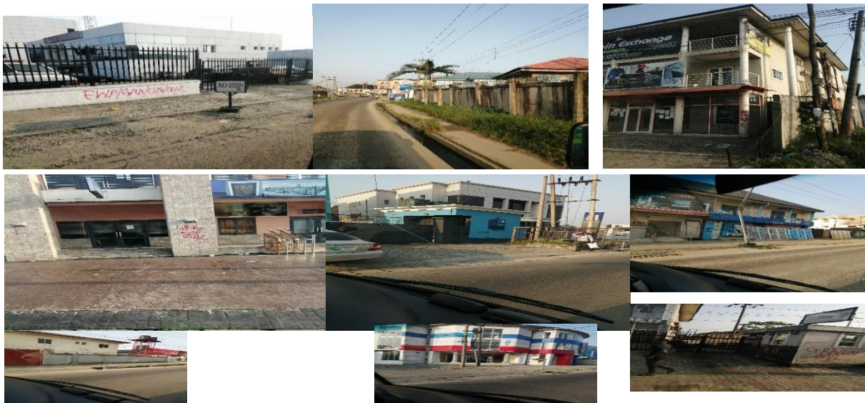
Plate 6.1: Some affected structures, marked for acquisition for the Flyover/road ROW
