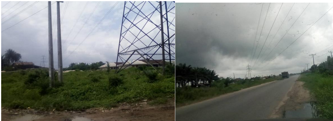
Plate 4.1 (a) RoW at Amukpe, Sapele TL and 4.1(b) T/L cutting through East West road near Ugheli Substation
