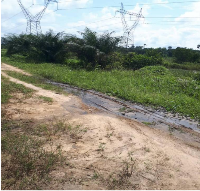
Plate 4.1 (c): Earth road from old Benin-Warri express road to TL by Oviri court community
