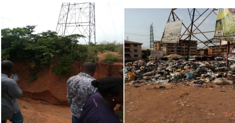
(A) Gully erosion sites at Ama Apu lfe (B) Dumpsite at tower (T1) at Ugwuagba Obosi,
