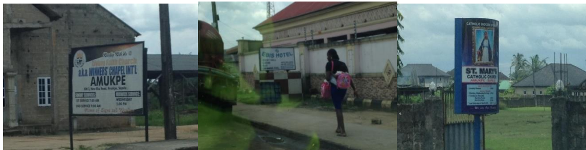
Plate 4.14: walling materials in the project area
