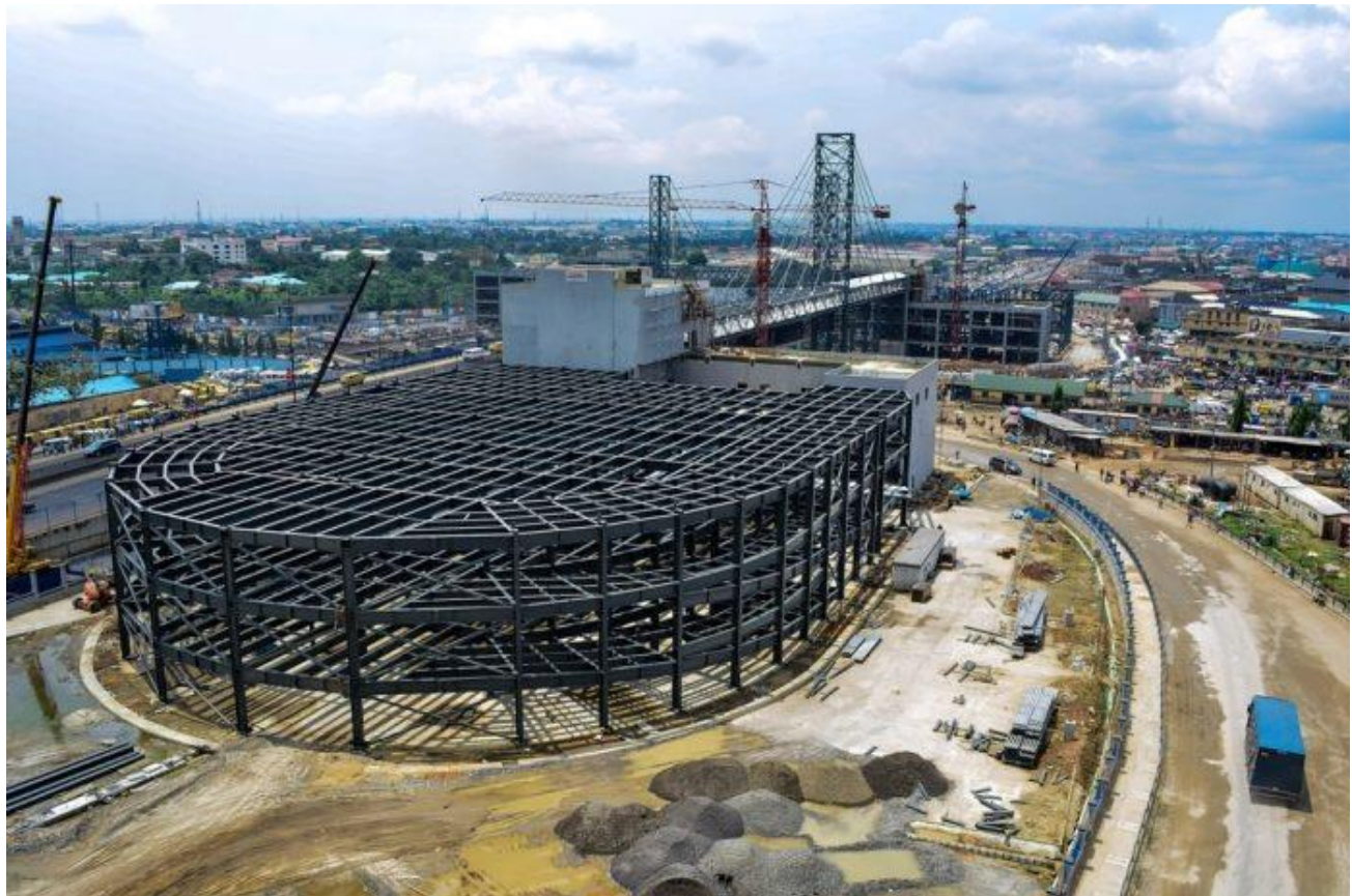
Plate 1.4: View of a typical transport interchange in Victoria Terminus in London, during construction activities
