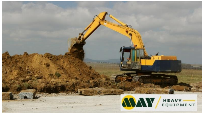
Plate 3.1: Typical excavator at work
