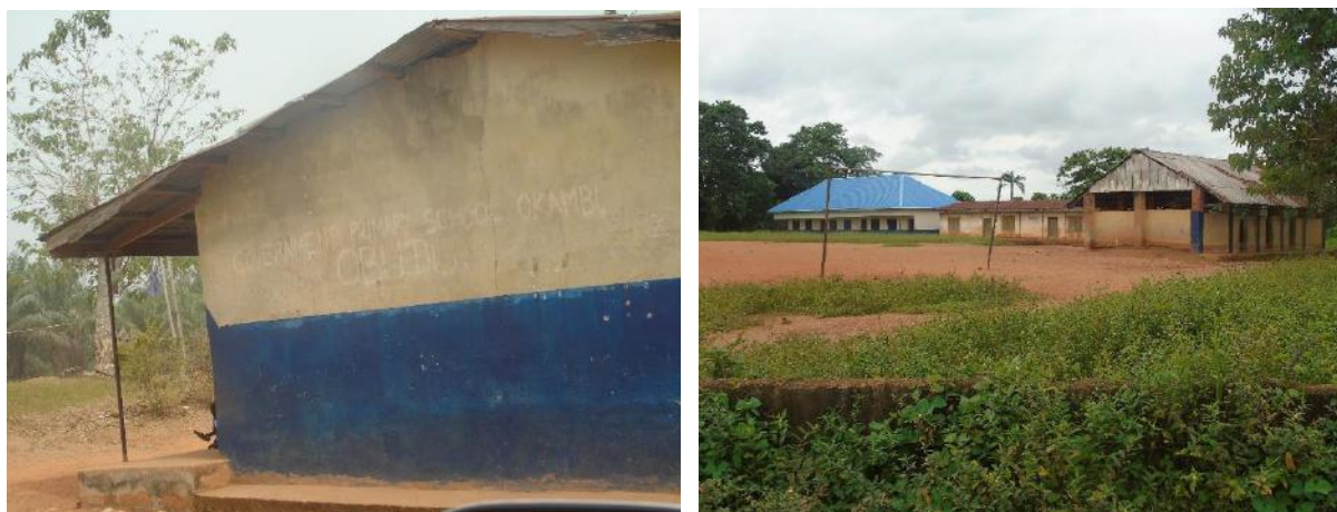
Plate 4.20: Old and newly renovated blocks of Primary School within Okambi community
