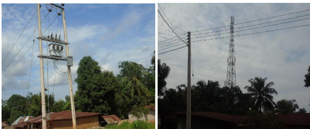
Plate 4.30: Electricity and telecommunication facilities across the host communities
