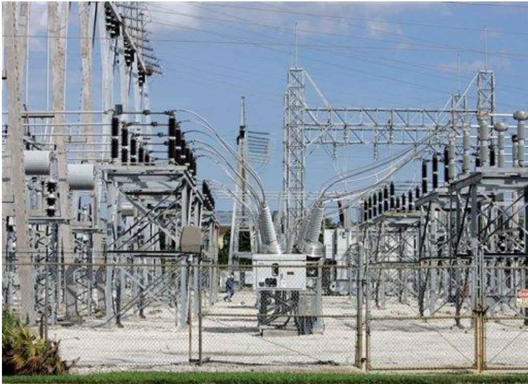
Figure 3.3.1a: A typical transmission substation showing switchgears
