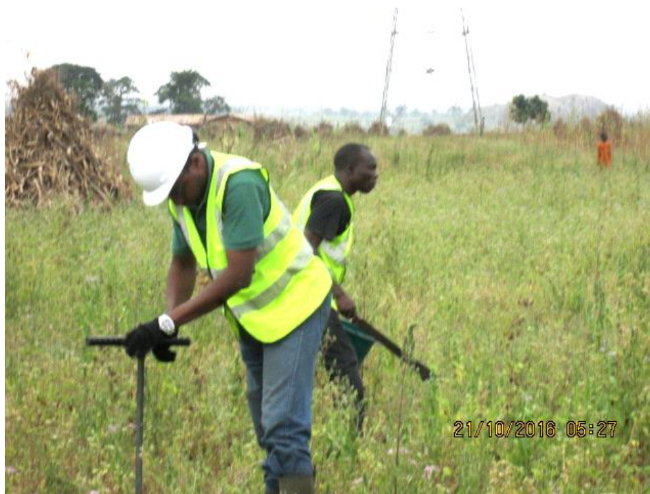
Plate 4.2.5.1: Collection of soil sample using auger at a sampling location
