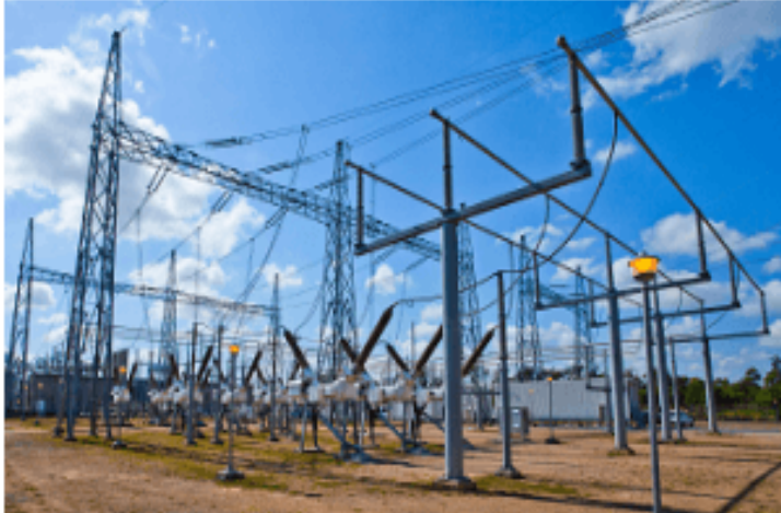
Plate 3.13: Picture of switchyard in a substation
