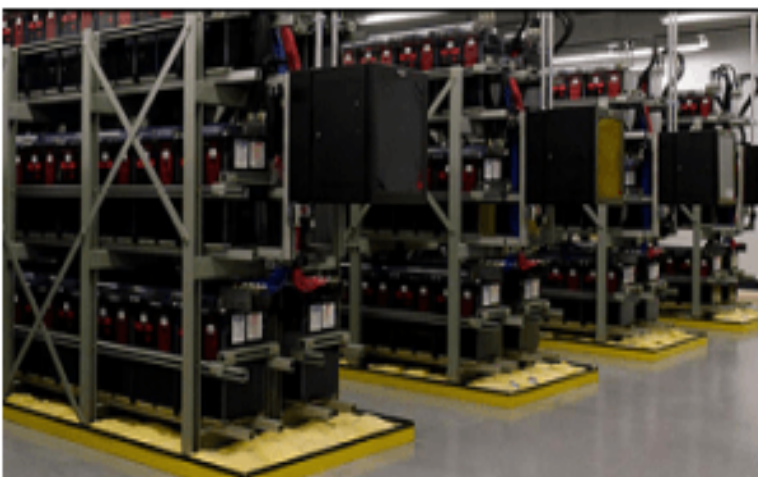
Plate 3.11: Picture of batteries in a substation
