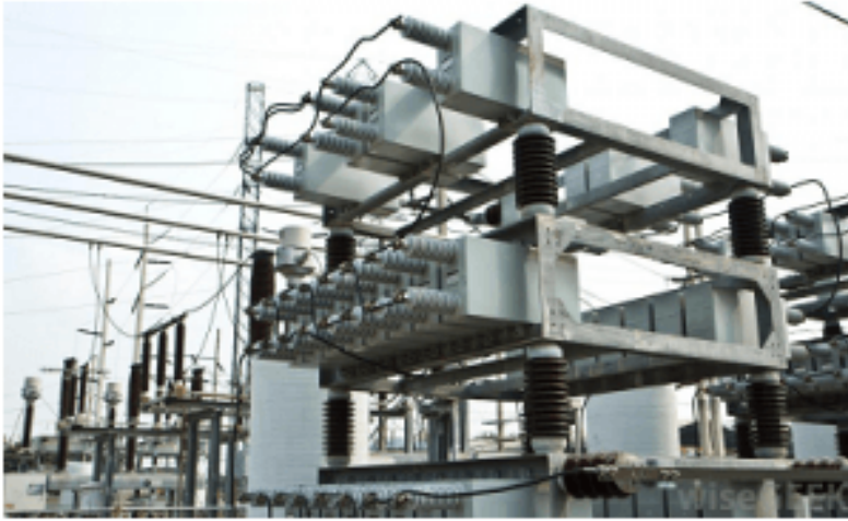
Plate 3.10: Picture of capacitor banks in a substation
