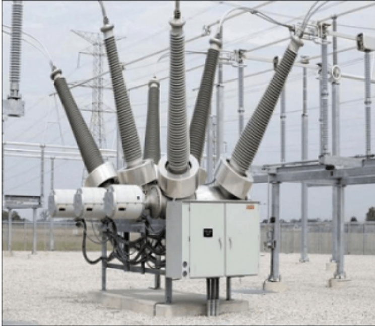
Plate 3.8: Picture of circuit breaker in a substation
