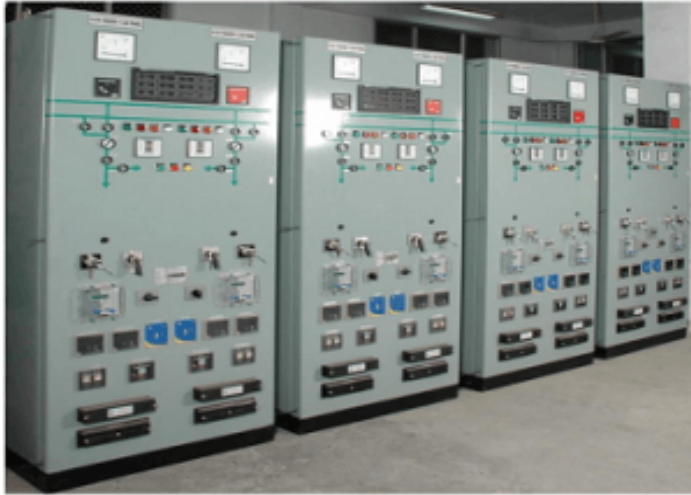
Plate 3.9: Picture of relays in a substation
