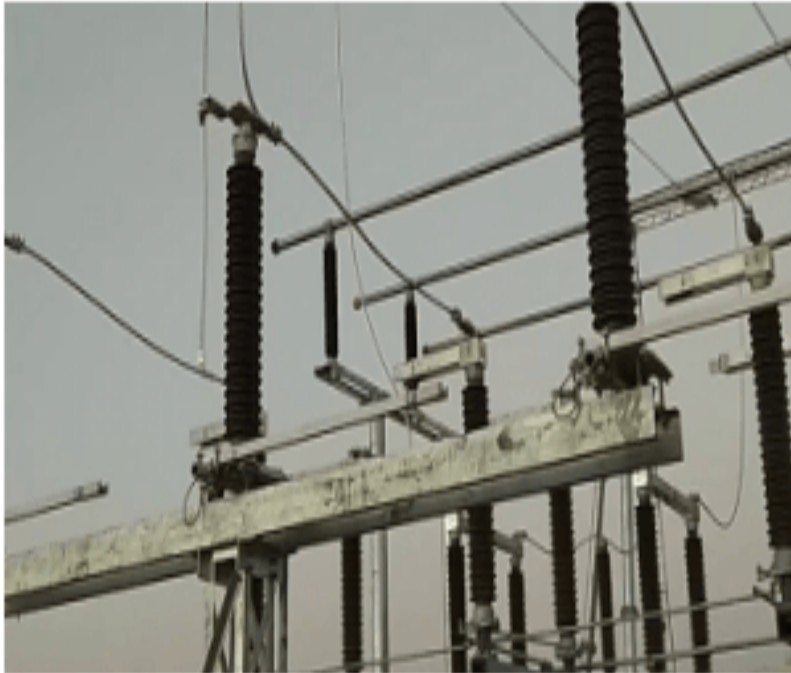
Plate 3.6: Picture of a typical busbar in a substation
