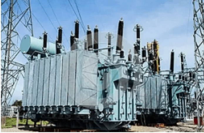
Plate 3.14: Picture of a Step-down Substation
