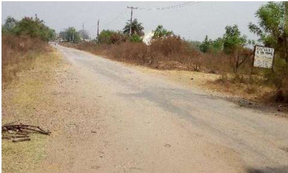
Plate 4.12a: Section of the main road leading to Ajaokuta
