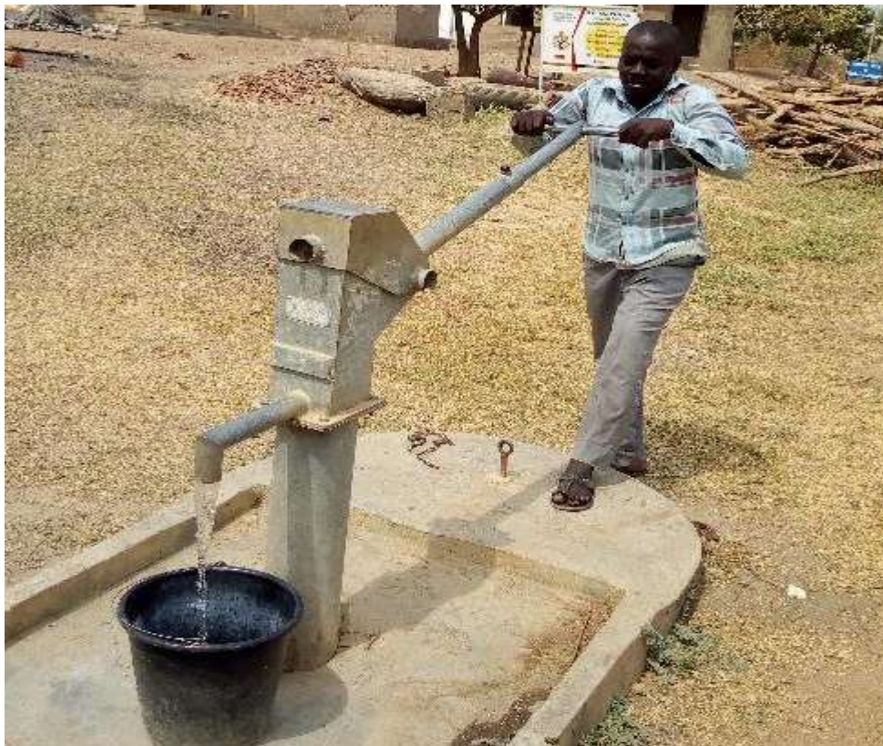
Plate 4.14: Manual borehole used in Ajaokuta community
