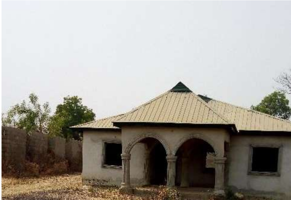
Plate 4.9b: A modern house under construction observed in Ajaokuta
