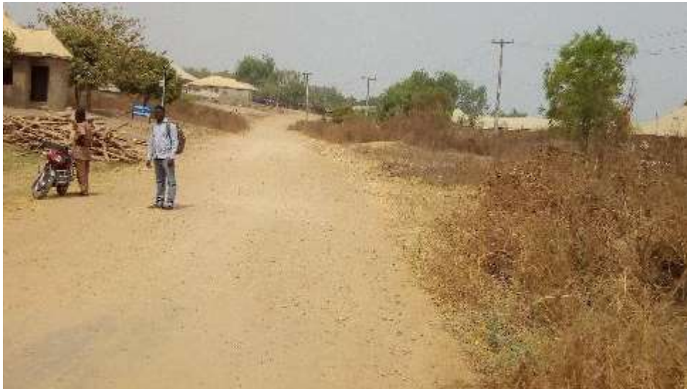
Plate 4.12b: Road section of a street in Ajaokuta
