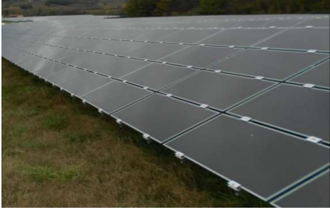
Figure 2.4: Typical appearance of Thin-Film CdTe panels
