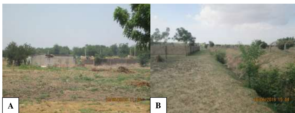
Plate 4.5: (a) Dilapidated structures within the Project site (b) a section of the temporary military trench on the site
