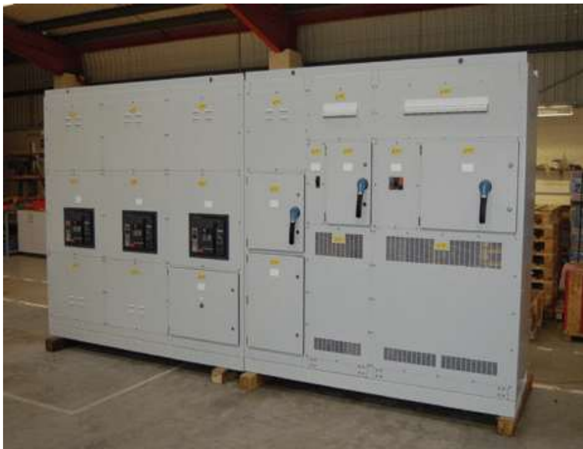
Plate 3.3: A typical low voltage switchgear cabinet
