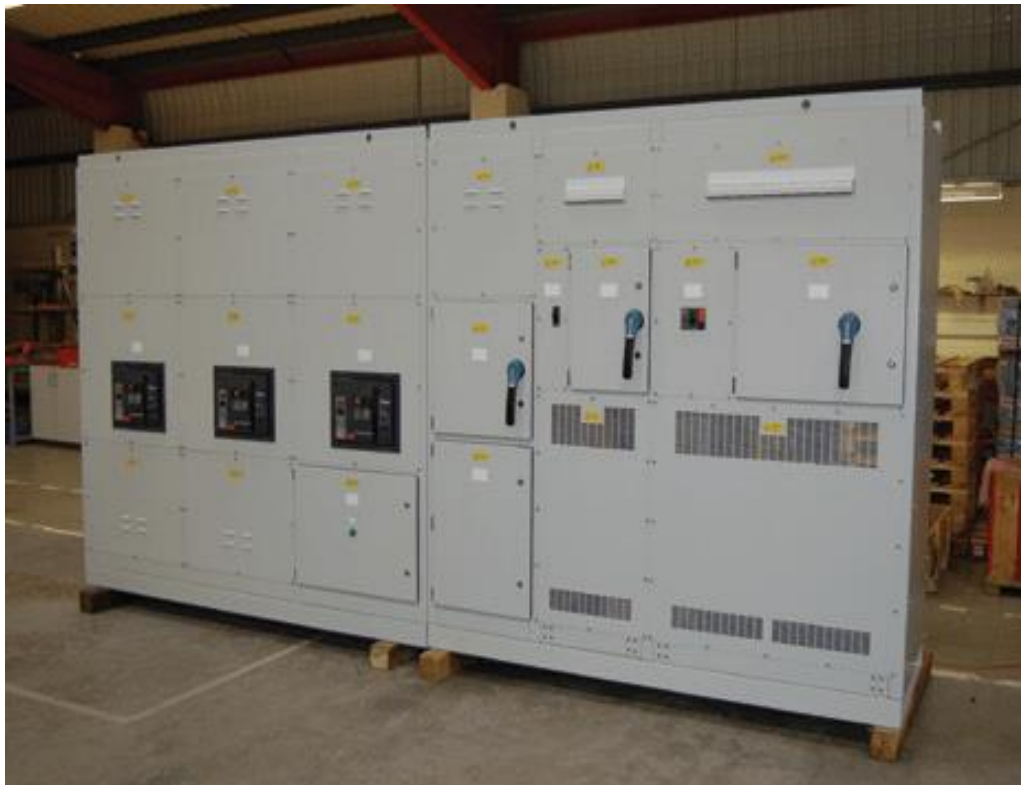
Plate 3.2: A typical low voltage switchgear cabinet
