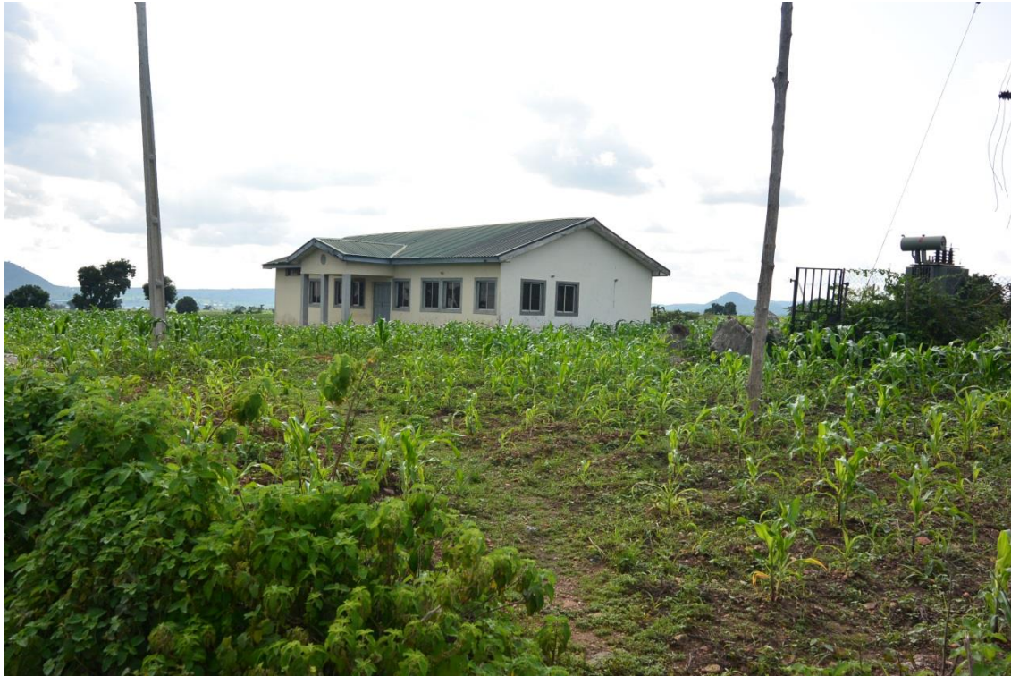
Plate 4.5: Unoccupied building observed on the site
