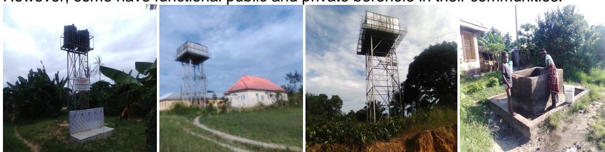
Plate 4.16: Functional borehole at Kwampa by Mary Remarkable Foundation and typical of non-functional boreholes by NDDC and hand dug well in Utapate Field communities.
