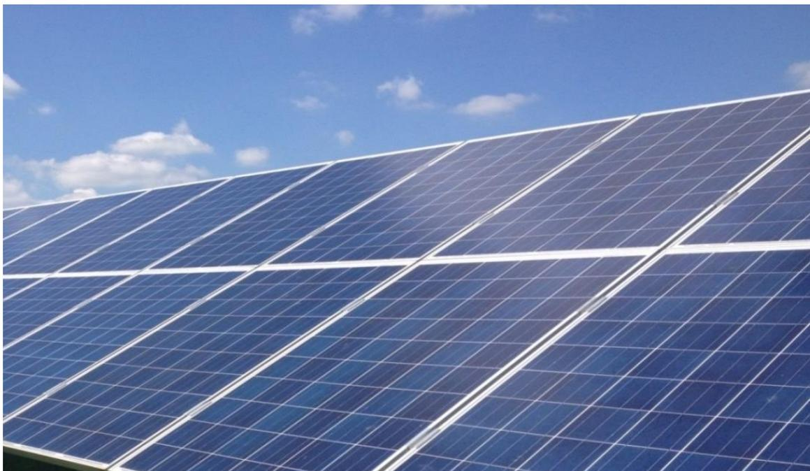
**Figure 2.3: Typical Appearance of Polycrystalline Silicon PV panels**
