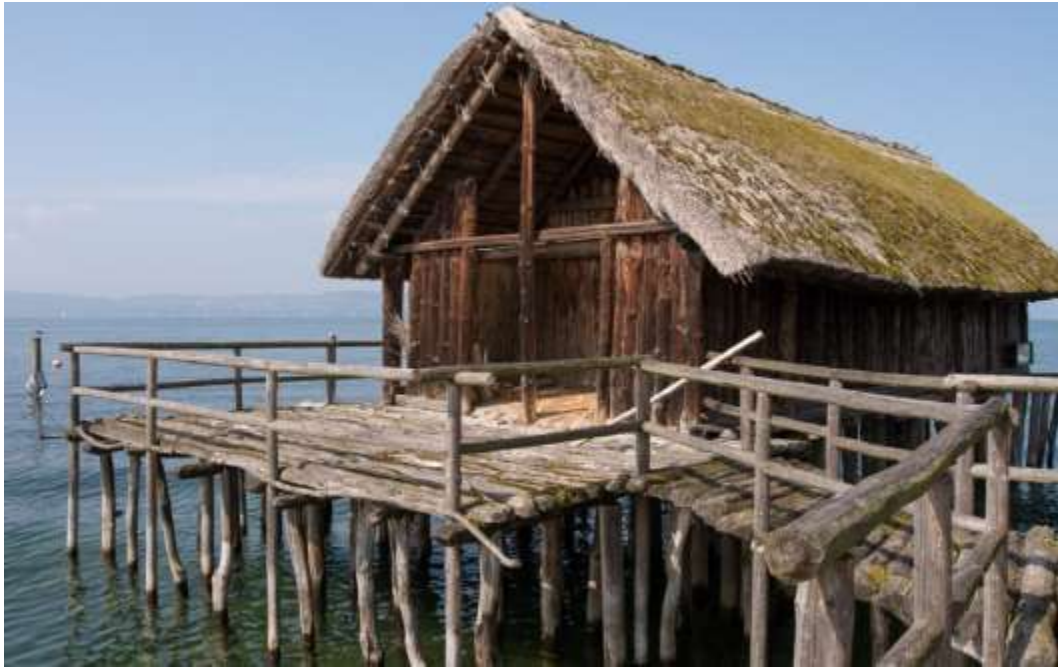
Plate 4.14: Raised building foundation in Araromi seaside
