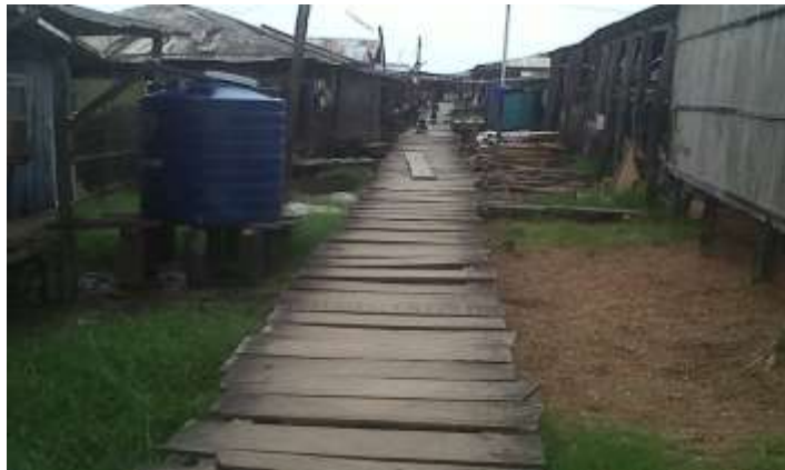
Plate 4.8: Wooden planks are the predominant construction materials in Aiyetoro
