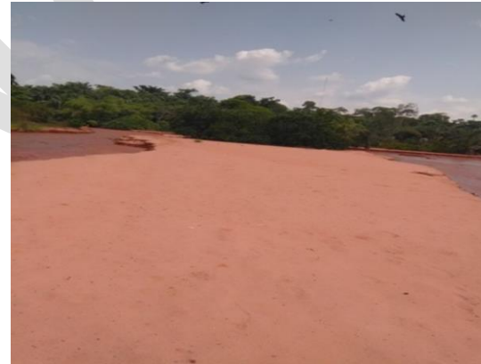
Obibia River (N 06° 14.453'; E 007° 04.498') Gully Outfall Area
