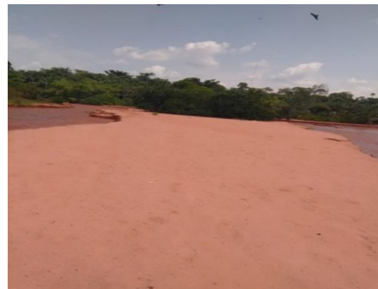
Obibia River - Erosion Outfall Area
