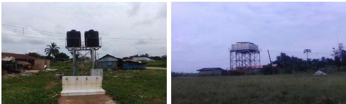
Plate 4.19: Showing functional Amnesty borehole water and non-functional Niger Delta Development Commission (NDDC) borehole water respectively
