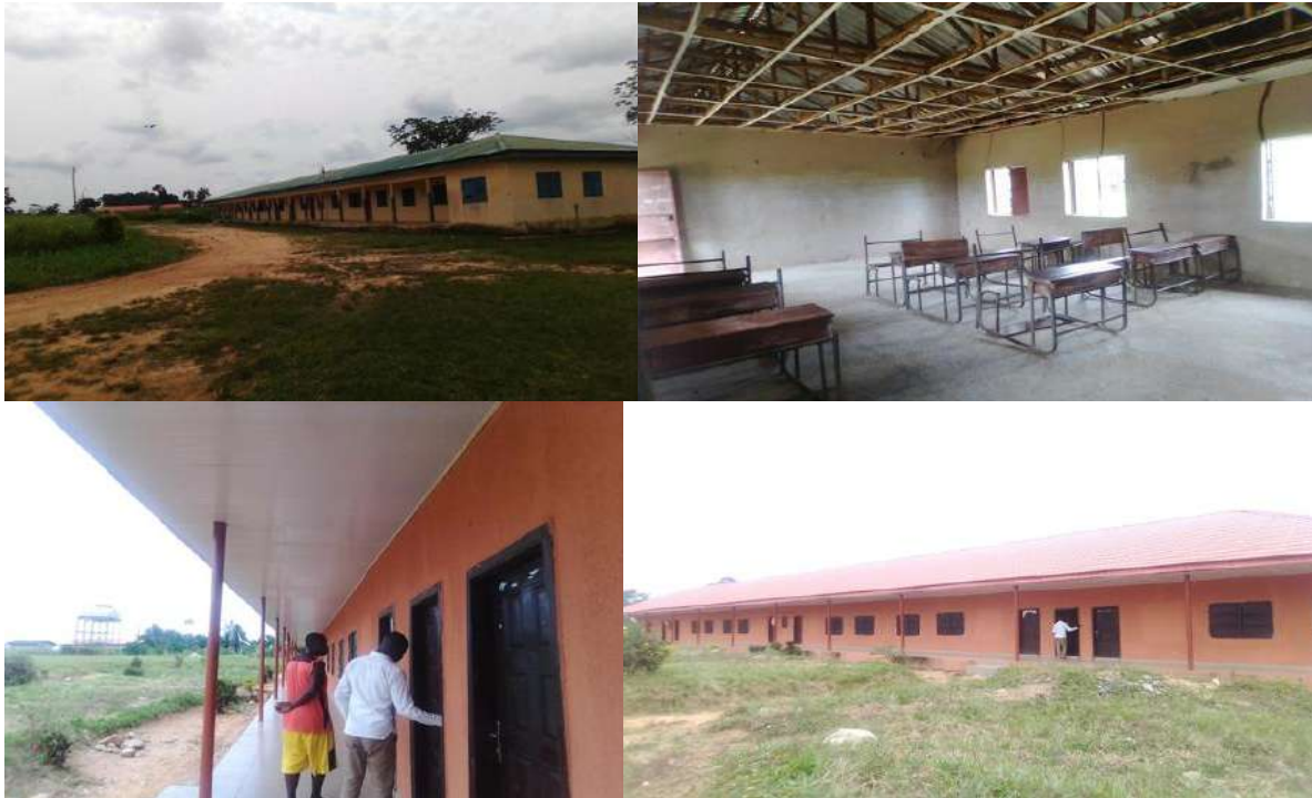
Plate 4.17: Showing primary and secondary school respectively in the community
