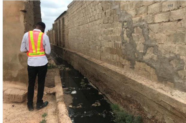
Figure 4: Section of Canal running through residence
