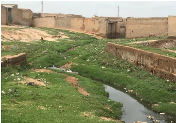
Figure 3: Section of Washed off canal
