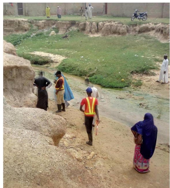
Figure 8: Erosion cutting off portions of land and structures close to eroded portions under threat
