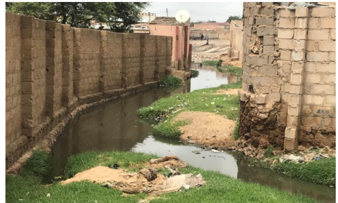
Figure 6: Section of the drainage canal in katsina
