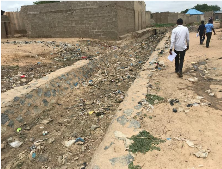
Figure 4: A Section of TsohowaTukari / Dan Tudu channel
