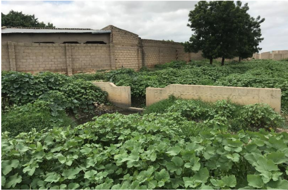
Figure 3: Section of the irrigation area overtaken by flood
