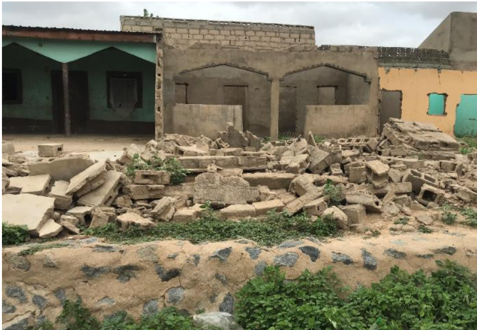
Figure 6: Structures damaged by the flood
