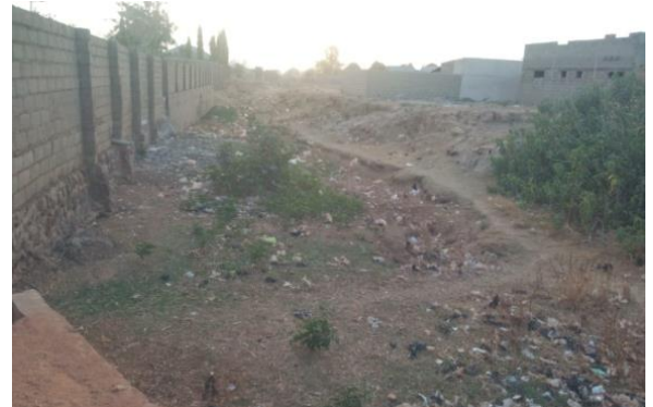
Figure 4: One of the Canal routes in Funtua with nearby structures
