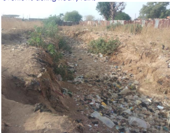
Figure 8: Solid waste issues inside the drainages with potential affected temporary structure along the side
