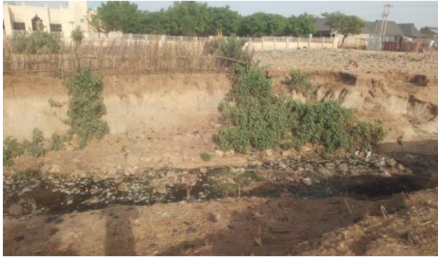
Figure 3: Washed off canal by flood in Funtua. Imminent danger of destruction for the adjoining walls as shown in the picture
