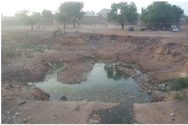
Figure 6: Pond caused by flood waters and harbours mosquitoes when water is stagnant. It overflows during heavy rains
