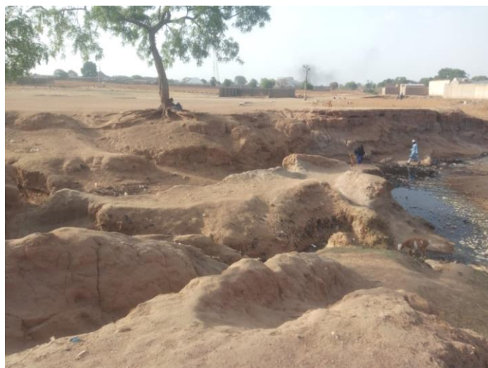
Figure 10: Erosion causing damage to peoples land and economic trees
