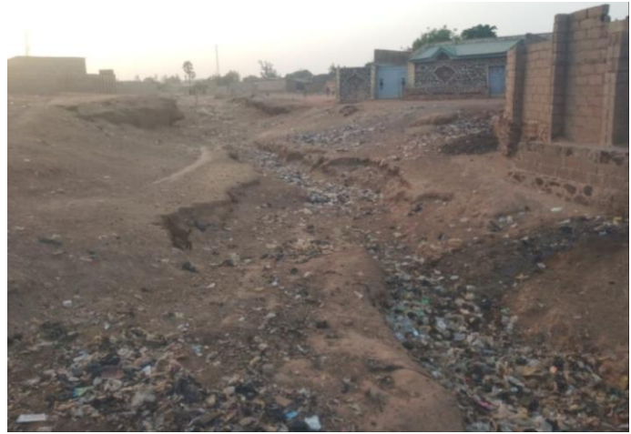
Figure 7: Drainage path with affected structures along the path
