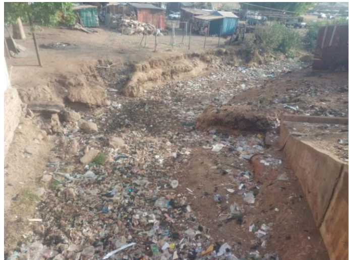
Figure 9: Drainage path with affected structures on either side. Management of solid waste is a major issue
