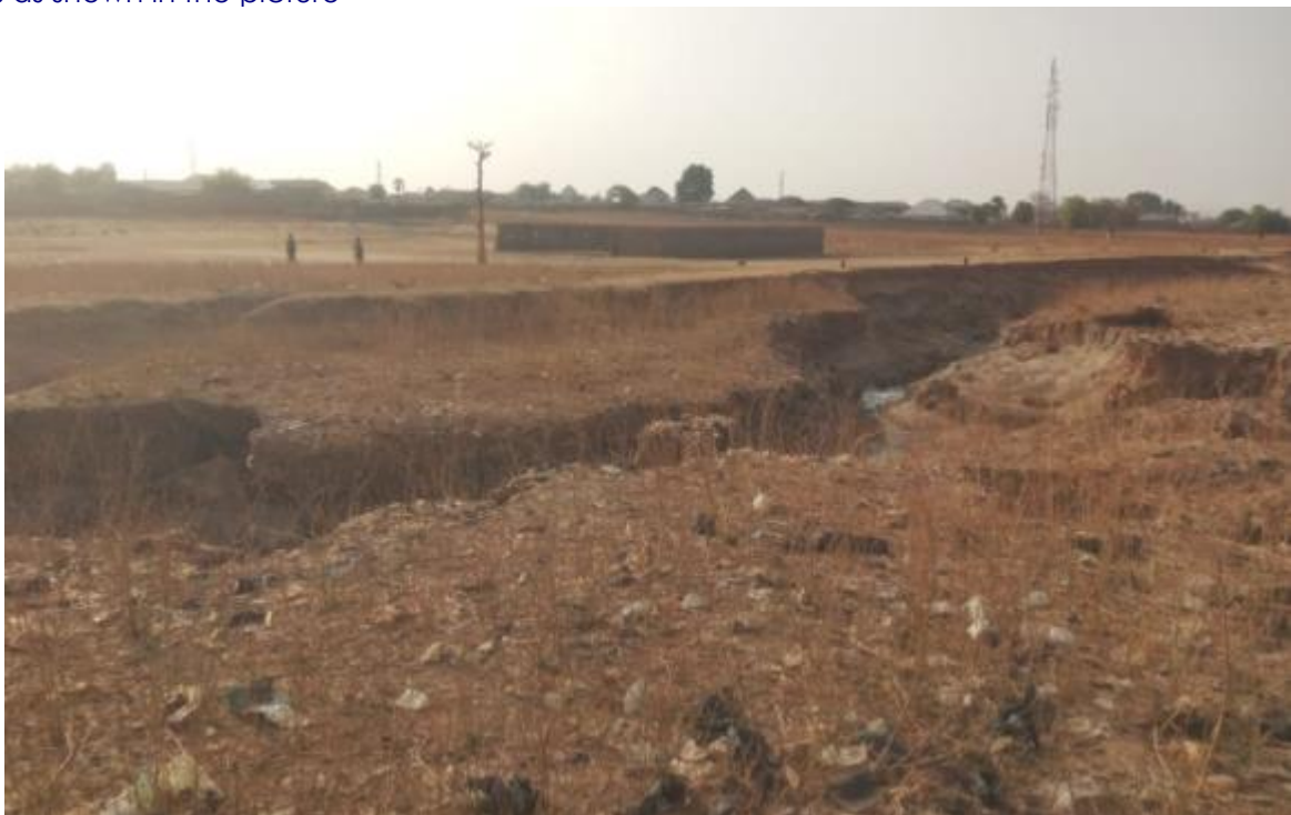
Figure 5: erosion resulting from wash off by flood in funtua
