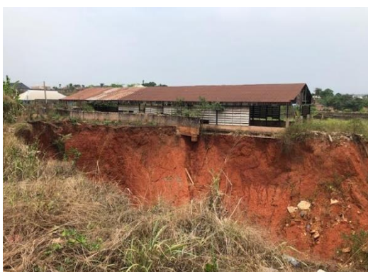
Figure 1 A Factory seriously threatened in between the main gully head and Finger (Iguosa Erosion RAP baseline studies March, 2020)
