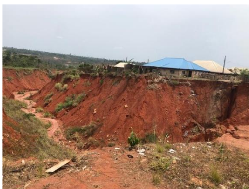
Figure 2 A Residential house close to the Gully mouth Finger (Iguosa Erosion RAP baseline studies March, 2020)
