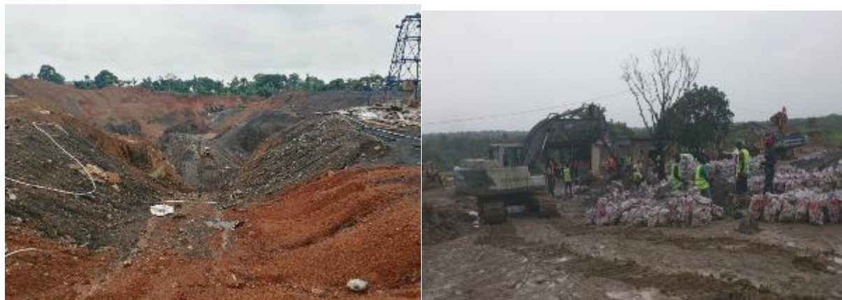
Figure 3.9: Small scale Mining of Lead and Zinc Ore at Jidech Mining Company, Mkpumakpatapa, Izzi LGA Ebonyi State
