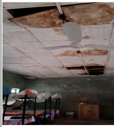
Plates 15: Rotting and Falling ceiling in a girl's hostel, walls and floors cracked and very old
