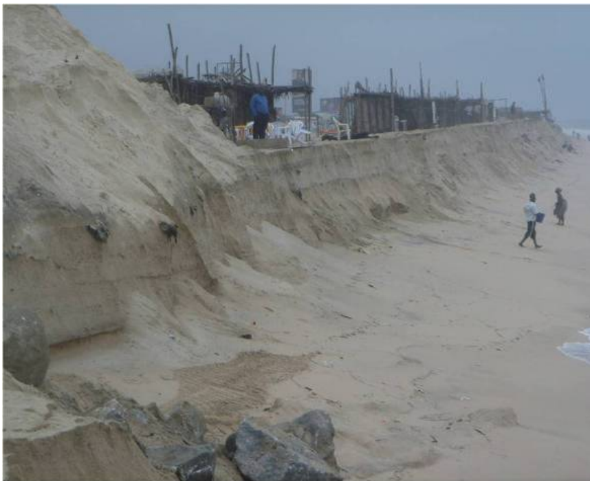
Plate 3.3 Erosion at Bar Beach c. 2006
