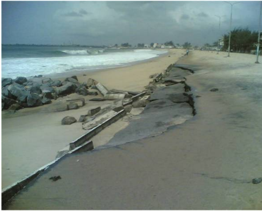
Plate 3.4 Erosion at Bar Beach c. 2006
