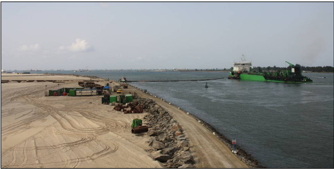
Plate 4.3 Example of sand pumping operations
