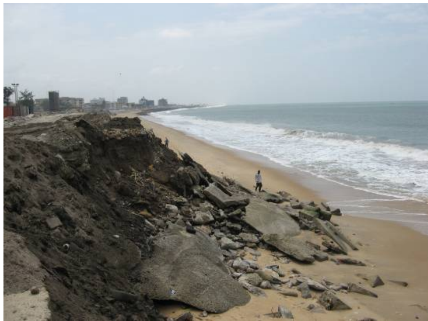
Plate 3.5 Erosion at Bar Beach c. 2006
