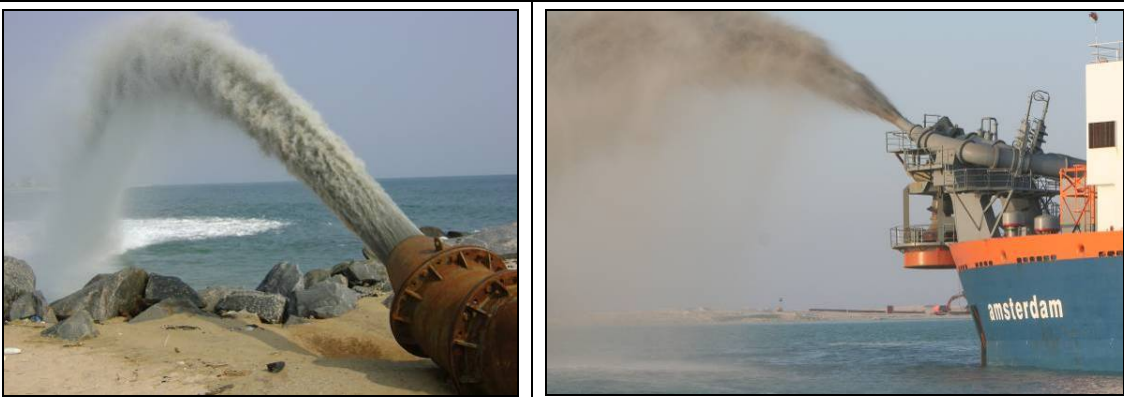
Plate 4.4 Sand placement via pipe (left) and rainbowing from dredging vessel (right)
