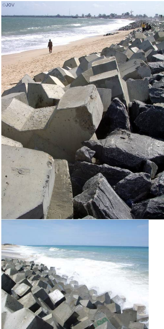
Plate 5.1 Recent Bar Beach shore protection works
