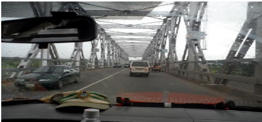
Plate 4.26 Niger Bridge at Onitsha
